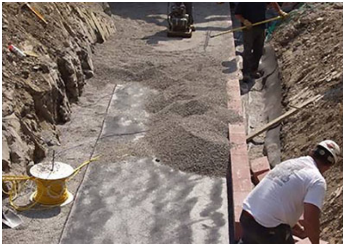
Geosynthetic reinforced soil bridge abutment under construction
