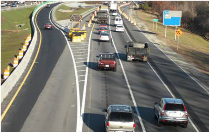
Typical traffic crossover utilized as part of the MassDOT Fast 14 project
