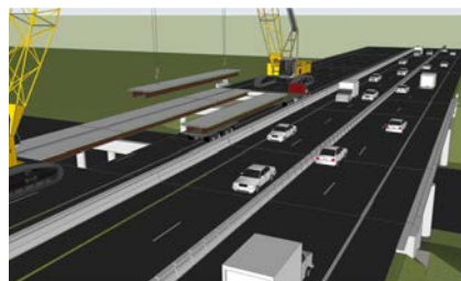
Artist's rendering of placement of prefabricated superstructure elements on the MassDOT Fast 14 project
