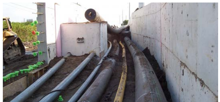
Utilities often need relocation or accommodation during construction projects in order to avoid disruption of services.
