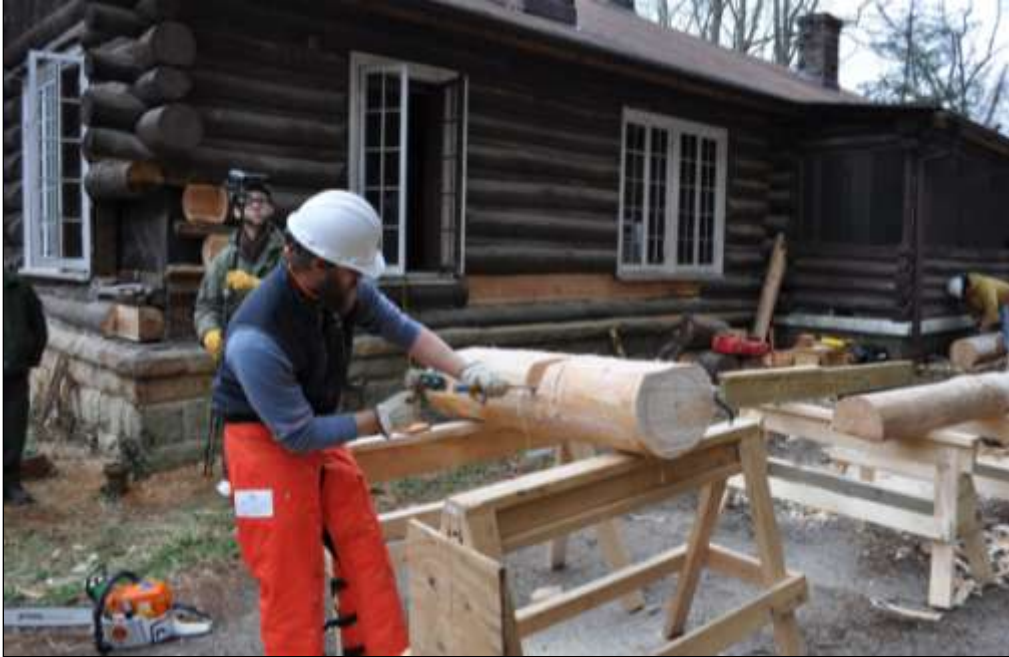
Ed FitzGerald films a worker notching a log during a workshop in Putney, KY.
