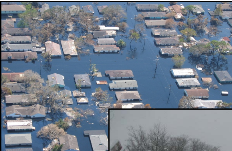
View of inundated areas in New Orleans following the breaking of levees surrounding the city as the result of Hurricane Katrina in 2005.
