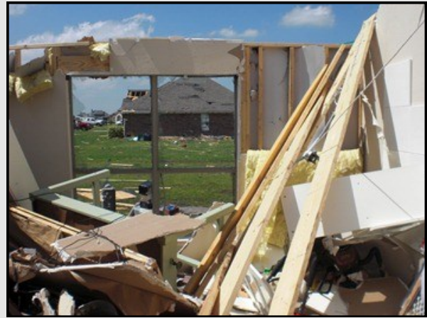
A picture of the room right outside the bathroom door. Extensive heavy debris like this was found in every room of Brooke's house, except for the internal bathroom.
