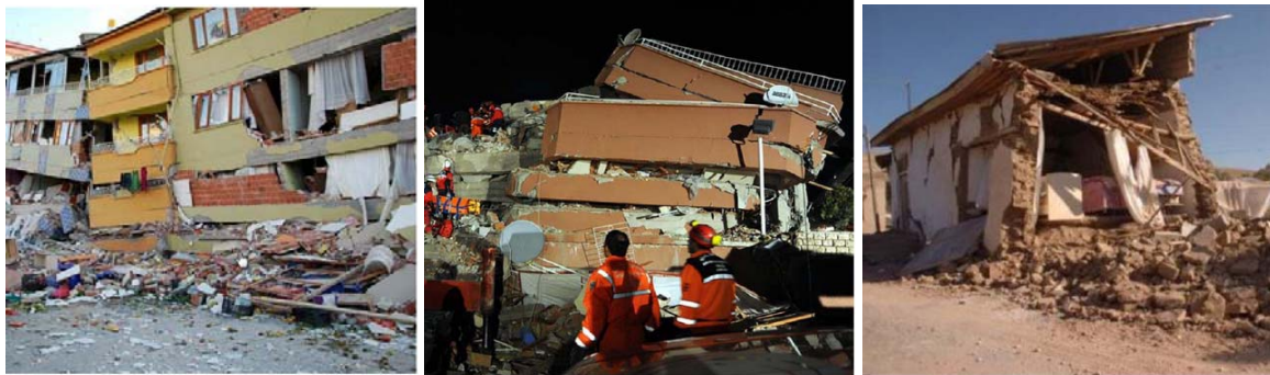
Figure 6: Soft storey collapse (left, gazetevatan.com); Pancake Collapse (central, fotogaleri.ntvmsnbc.com); Rural damage (right, gazetevatan.com)
