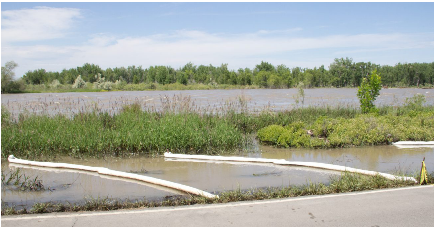
Booms along the Yellowstone River to capture spilled oil
