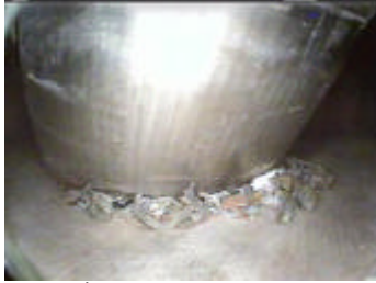
Figure 9 - CRDMP No. 78 Debris In Examination Area (As Found)
