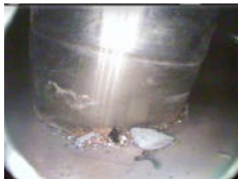
Figure 3 - CRDMP No. 33 Debris In Examination Area (As Found)
