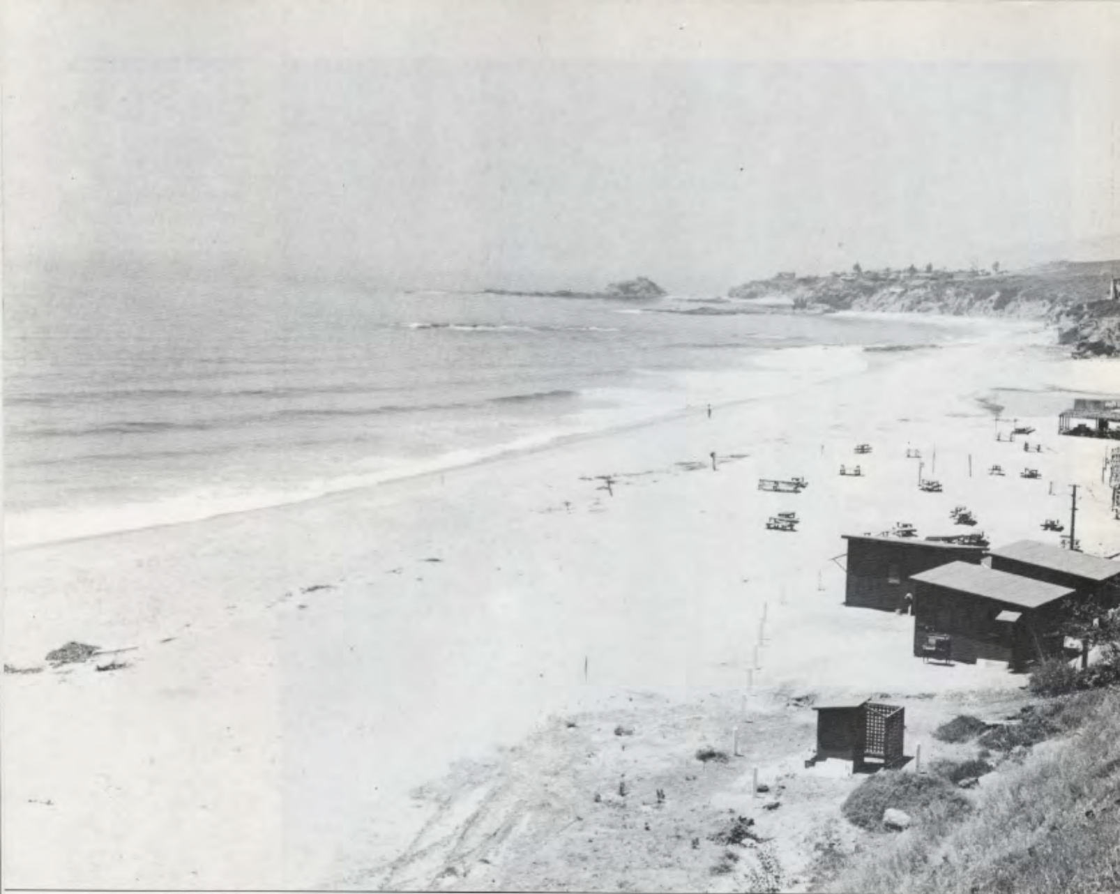
Above: Many Coast Guard Stations were located in out of the way locations.
