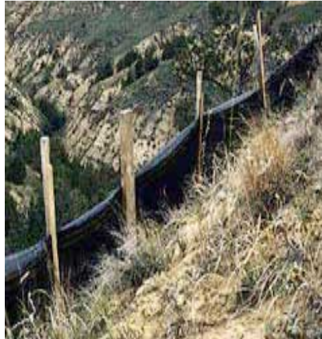
Sediment fences such as this are used to control erosion, trap large materials, filter sediment from rainwater, and slow runoff. Click on image for larger view.
