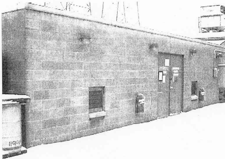
Photo 9. SAPS water treatment consumables building
