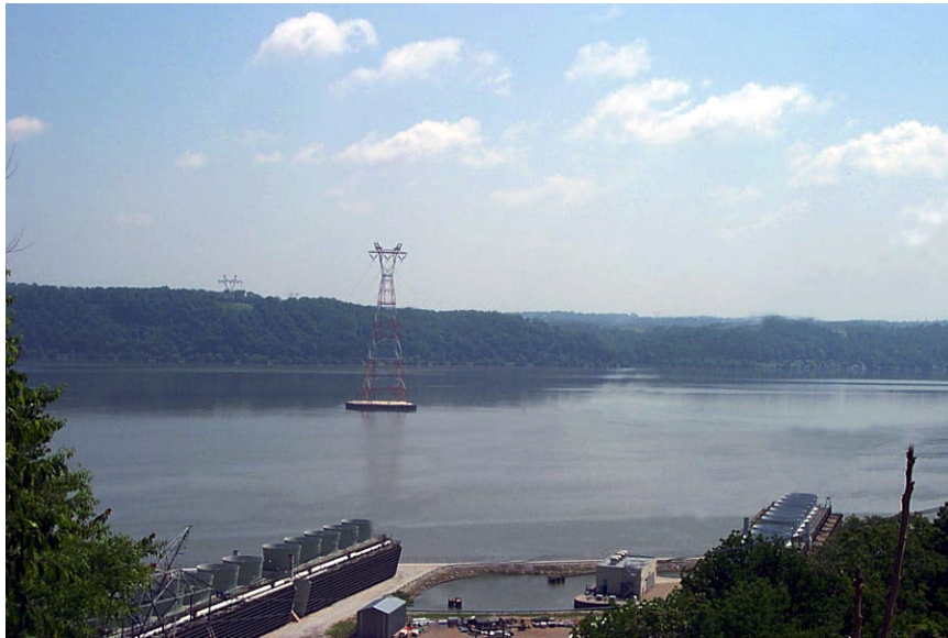
The 500-kV Peach Bottom-to-Keeney line crosses the Susquehanna River at PBAPS.
