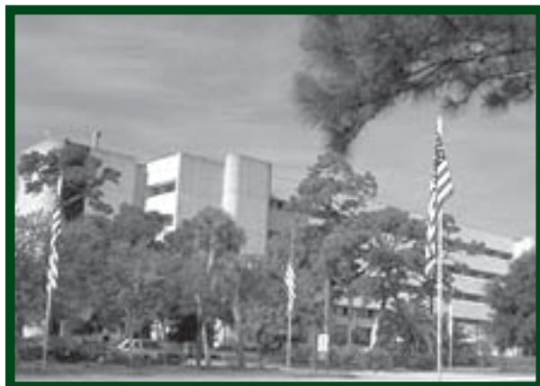
VA Medical Center Bay Pines, FL
