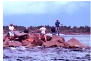
A jetty protecting the shore line. (Photo: NOAA)
