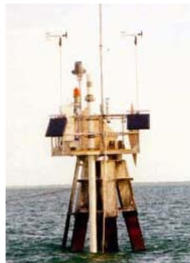
Seakeys stations transmit real-time data. (Photo: NOAA)
