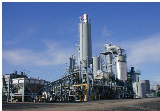
The kiln in Bayonne, New Jersey
