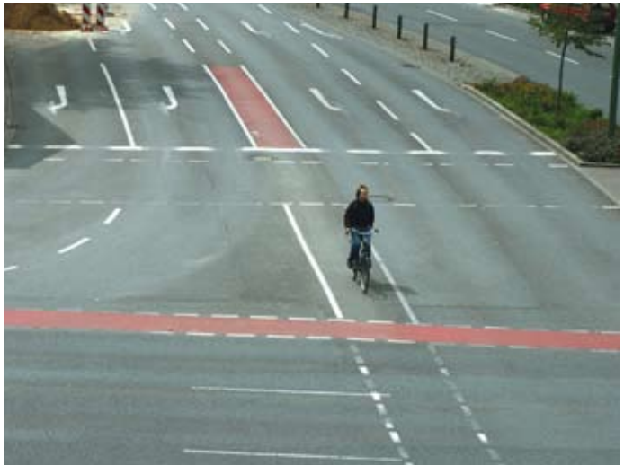
Figure 29. Dashed bike lane provides guidance through a wide intersection in Osnabrück, Germany. 6
