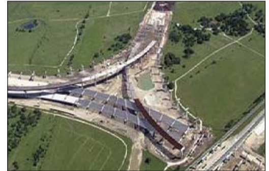
An aerial view of the Texas Turnpike
