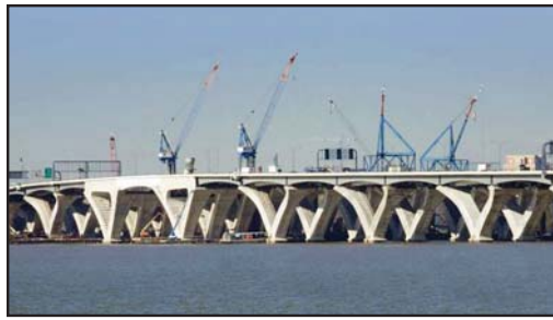
The Woodrow Wilson Bridge is a major project in the Washington, DC, metropolitan area.
