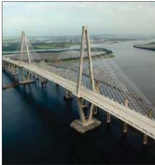
An aerial view of Cooper River Bridge, Charleston, SC
