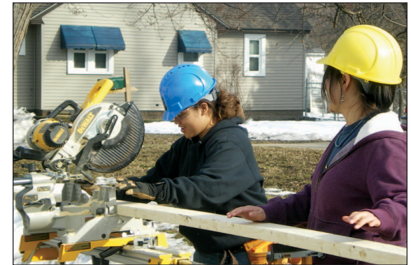
Participants cutting studs for new second floor.
