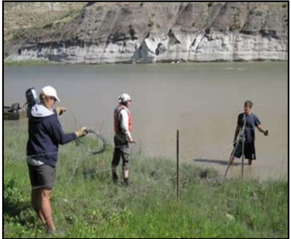
BLM staff extending a wing of riparian enclosure into the Missouri River
