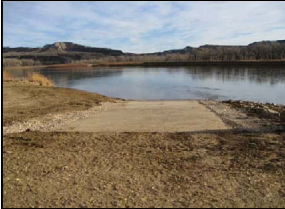
Judith Landing boat ramp – completed in October 2010
