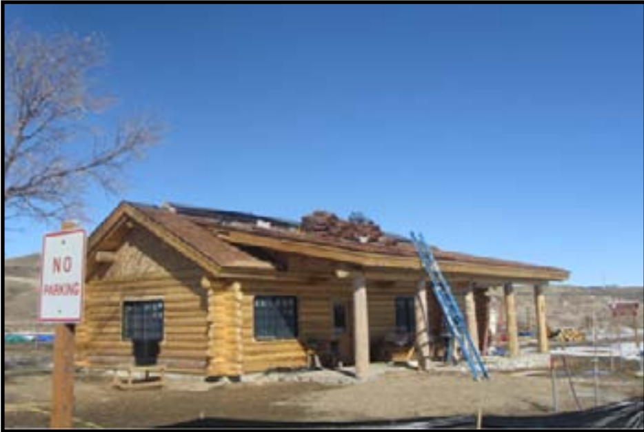
Coal Banks Landing contact station under construction
