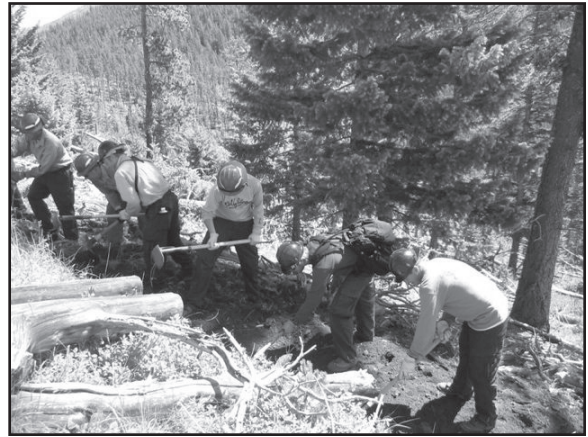
Firefighters from the Central Montana Fire Zone rolled up their sleeves and built trail like there was no tomorrow. BLM photo
