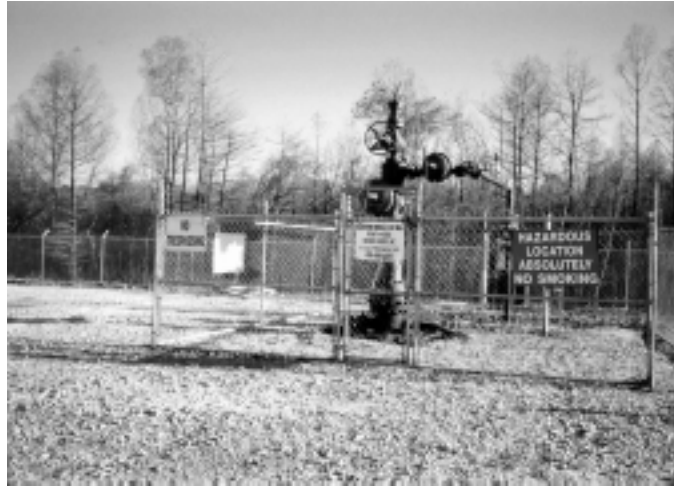
Example of well-maintained production operation near the Beaumont Unit, Big Thicket National Preserve, Texas.
