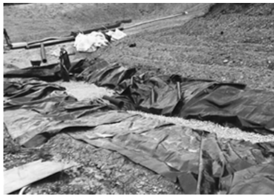
Anoxic limestone drains were constructed to raise pH of mine spoil effluent. This photo shows the drains during construction.
