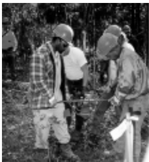
Hand-drilling seismic shot-holes for 3D survey in Big Thicket National Preserve, Texas.
