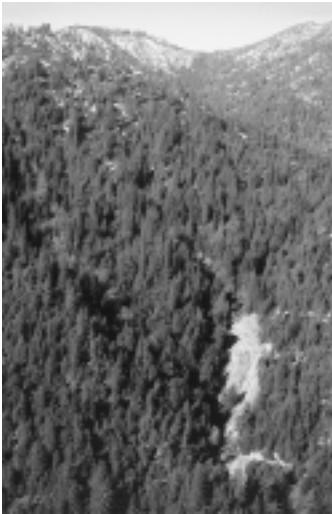
This debris flow originated at an abandoned logging road in Whiskeytown NRA during the 1997 New Year's storm. The road fill became saturated, "out of balance" with adjacent stable landforms, and consequently failed.
