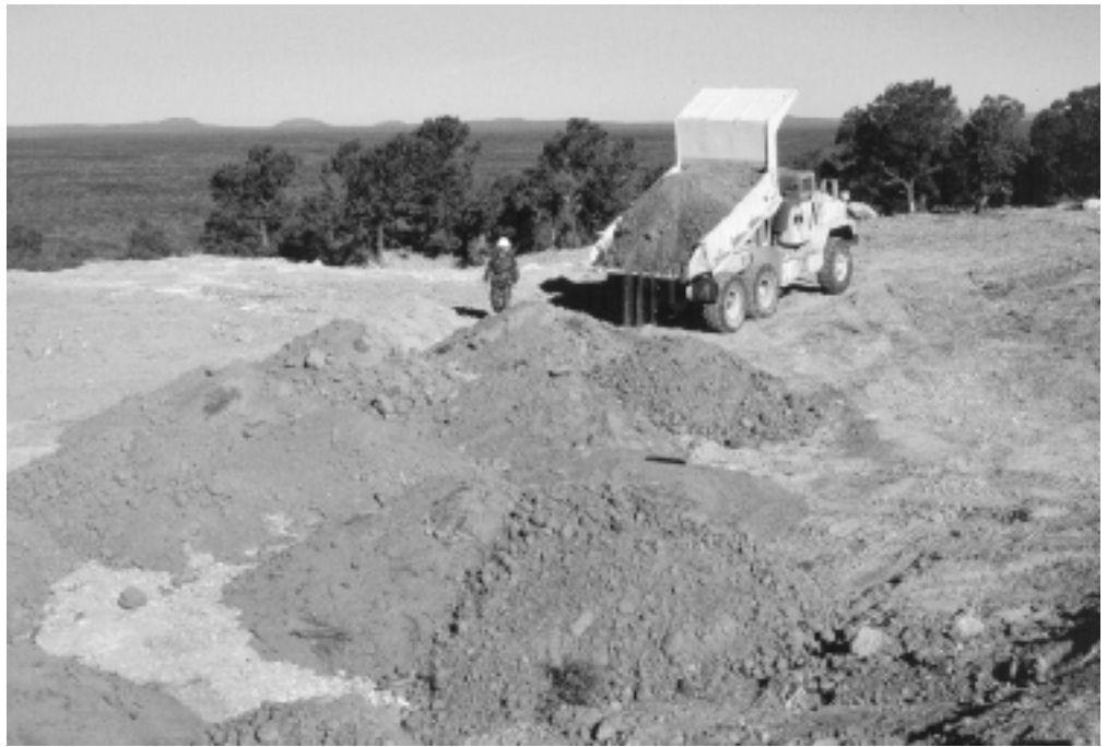
After establishment of final surface contours, topsoil was placed, and then graded, to provide the best possible conditions for revegetation at El Malpais.
