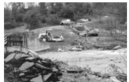
The debris flow also destroyed three bridges within the park.
