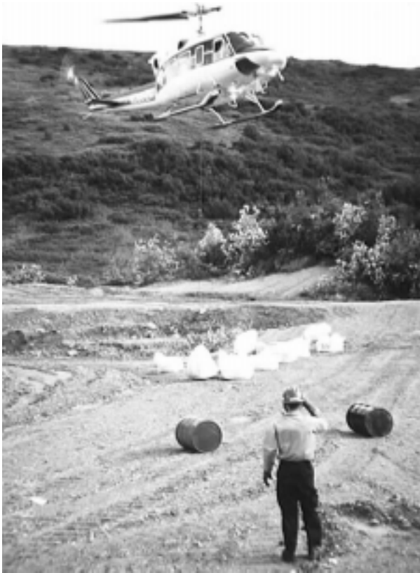
Limited access to the Slate Creek site required the park to transport lime and other supplies by helicopter. Lime was applied to acid generating spoil to increase pH at Denali National Park & Preserve.
