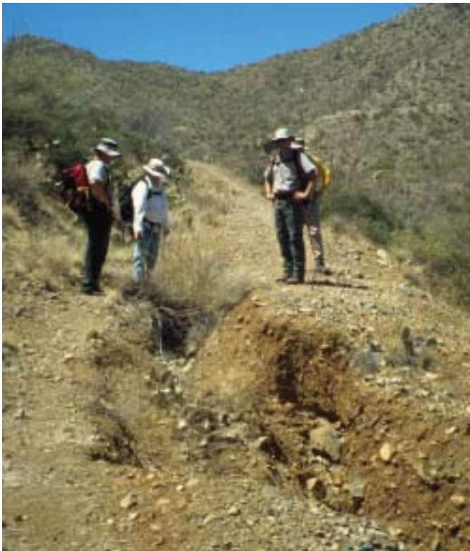
Roads divert surface flow and cause accelerated erosion, even in arid environments such as Saguaro NP.
