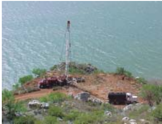
Plugging of an oil and gas well at Lake Meredith NRA in May 2001.
