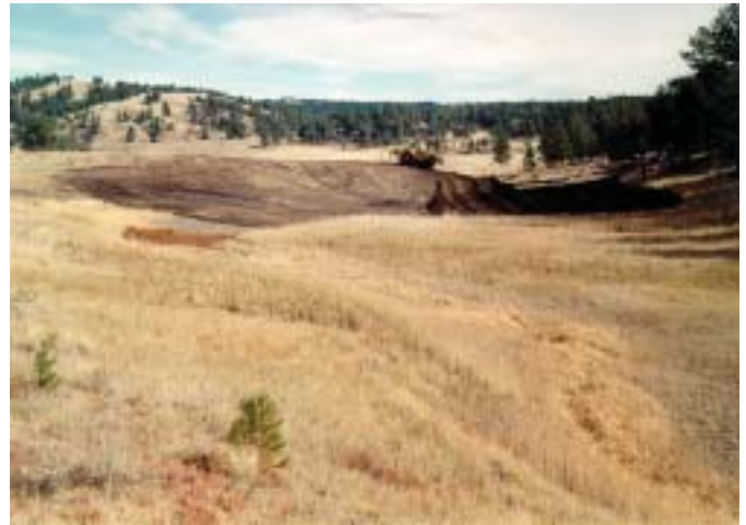
Heavy equipment, similar to that used to construct the dam, is used to reestablish naturally functioning landforms.
