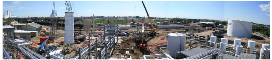
ClearFuels Rentech Integrated Biorefinery Construction - July 2011
