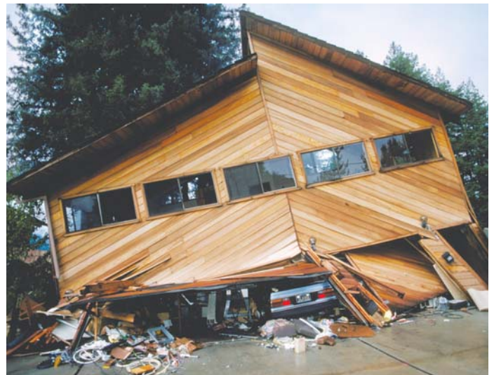
This home in the Santa Cruz Mountains, California, collapsed in the 1989 magnitude 6.9 Loma Prieta earthquake (USGS photo).
