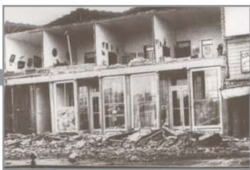
1906—Damage in Healdsburg
