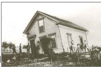
1868—Damage in Hayward
