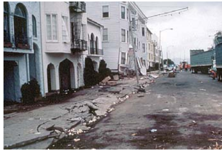
Liquefaction —Earthquake shaking can cause soils to behave like a liquid and lose their ability to support structures. Liquefaction often causes buried gas and water lines to break. The highest hazard is in low-lying areas where there are loose, sandy soils or poorly compacted artificial fill. This photo shows liquefaction-related damage in the Marina District of San Francisco following the 1989 magnitude 6.9 Loma Prieta earthquake (USGS photo).
