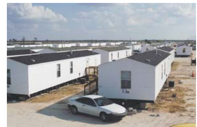
FEMA mobile homes being set up in Port Charlotte, Florida, to provide temporary housing for victims of Hurricane Charley (August 2004). Nearly a year after the storm, these trailers were still being used. (FEMA photo.)
