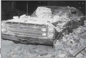
1969—Damage in Santa Rosa
