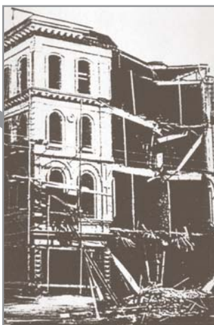
1865—Damage in San Francisco
