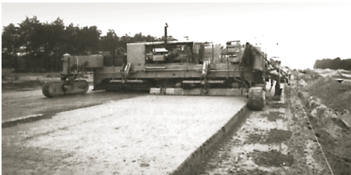
Figure 33. Slipform paving in Belgium began around 1970.
