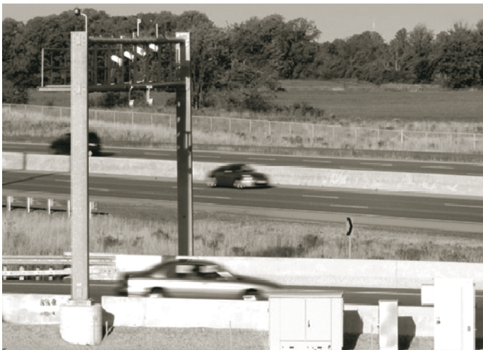
Figure 4. Vehicle passes under electronic sensors on gantry at on-ramp to 407 ETR.
