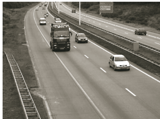
Figure 37. Jointed concrete motorway pavement in the Netherlands with full-width outer shoulder as emergency lane.
