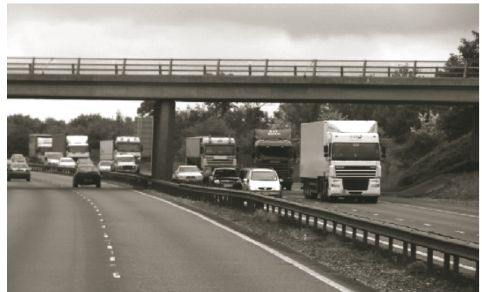
Figure 17. Thin asphalt surfacing mandated on concrete roads in England.
