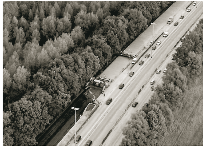
Figure 44. CRC overlay construction on E40/A10 in Belgium.
