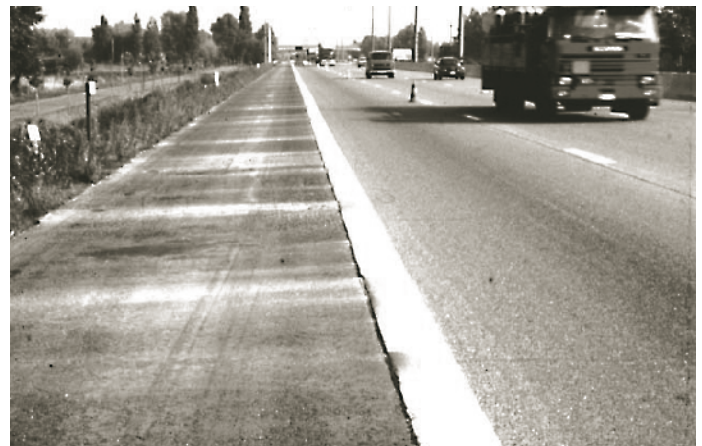
Figure 26. Pumping of fines from lean concrete base under Belgian CRCP built between 1977 and 1991.
