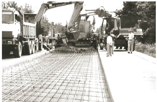
Figure 41. CRC inlay construction in Belgium.
