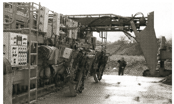
Figure 29. Dowel and tie bar inserters on back of front paver for two-lift paving in Austria.
