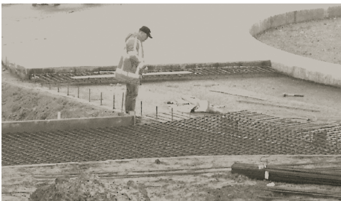
Figure 34. CRCP roundabout construction in Belgium.
