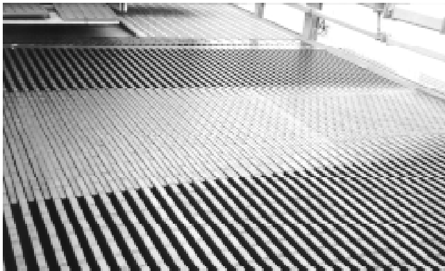
Figure 18. Riding surface of the expansion joint on the Akashi-Kaikyo Bridge.
