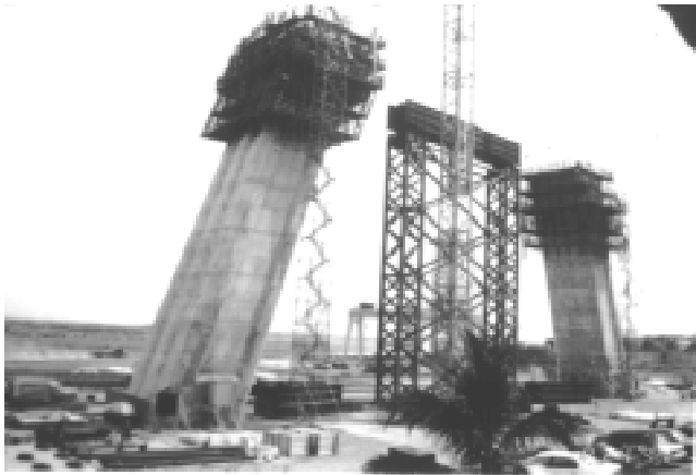
Figure 13. Kao-Ping River Bridge under construction.
