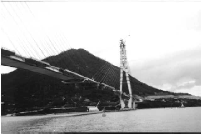
Figure 7. Tataro Bridge under construction
