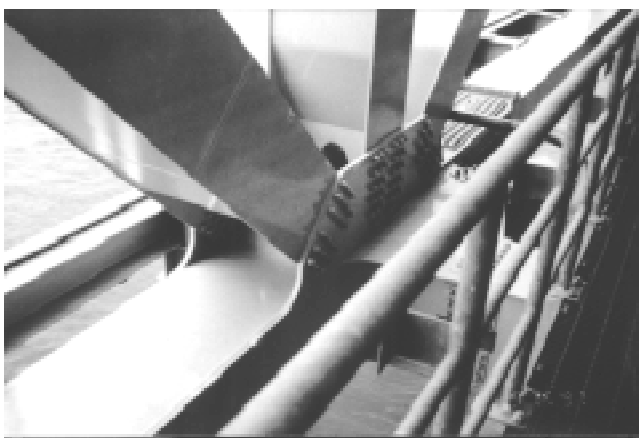
Figure 28. End connection of tapered members.
