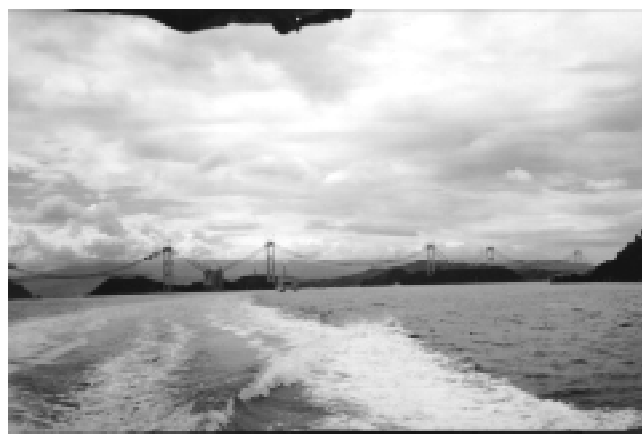
Figure 5. Kurushima Bridges under construction.
