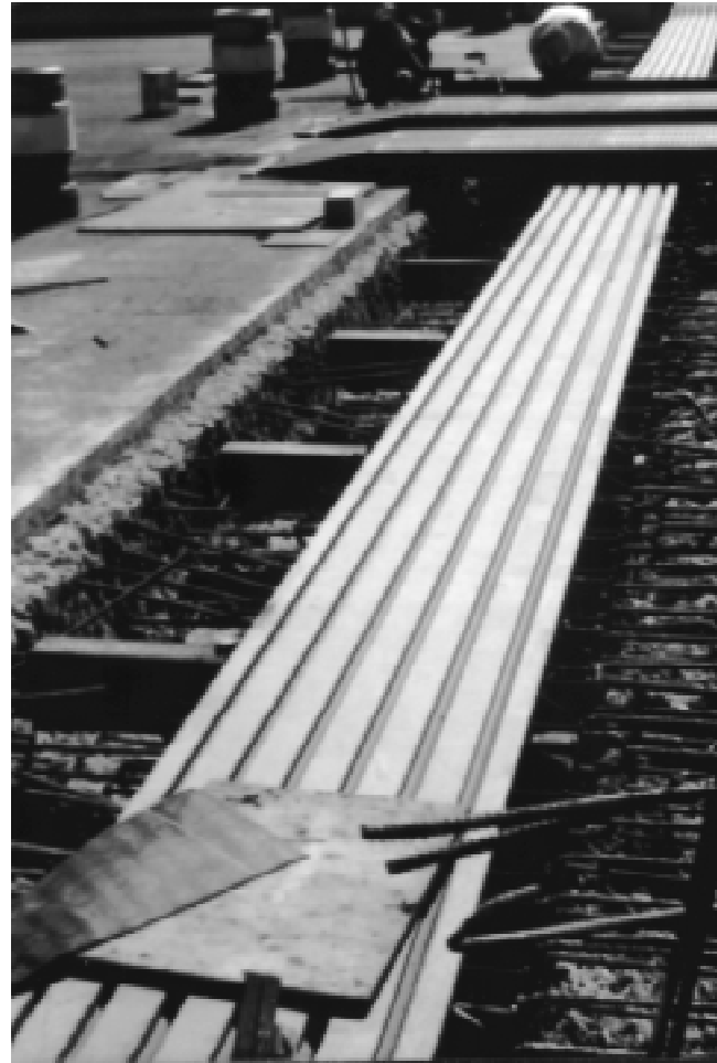
Figure 10. Installation of expansion joint on Kimp'o Grand Bridge.
