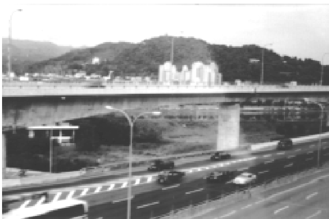
Figure 15. Hsichih-Wuku widening project.
