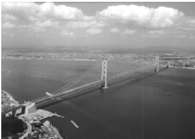
Figure 3. Akashi-Kaikyo Bridge (Photo by HSBA).
