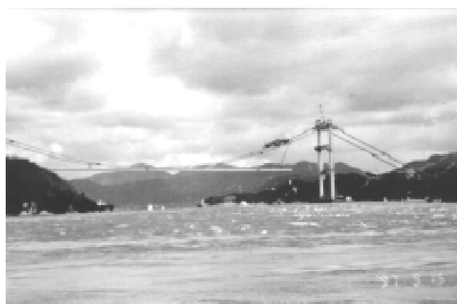
Figure 6. Kurushima 1 under construction.
