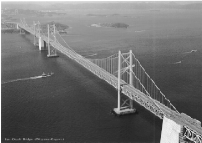
Figure 2. Suspension bridges on the Kojima-Sakaide Route (Photo by HSBA).
