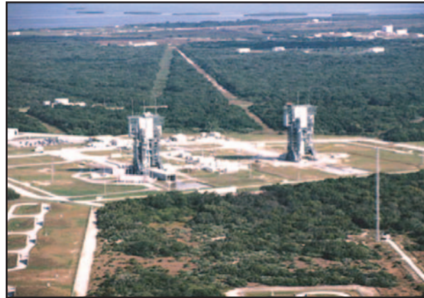
Cape Canaveral Air Force Station
