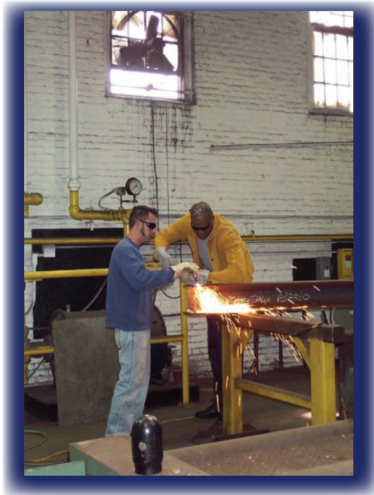
Steel Fabrication - Capco Steel
