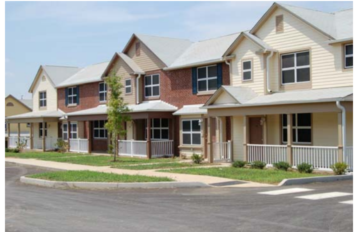
KHDC's Lonsdale Development. This is a renovated 1951 building. KHDC did different façade treatments to break up the "barracks look."
