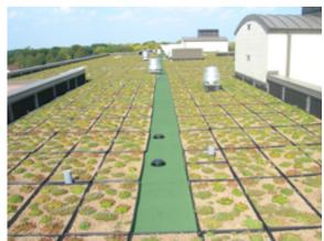
A green roof reduces the amount of heat the roof absorbs and reflects in summertime—a cause of poor air quality in many dense urban areas.
