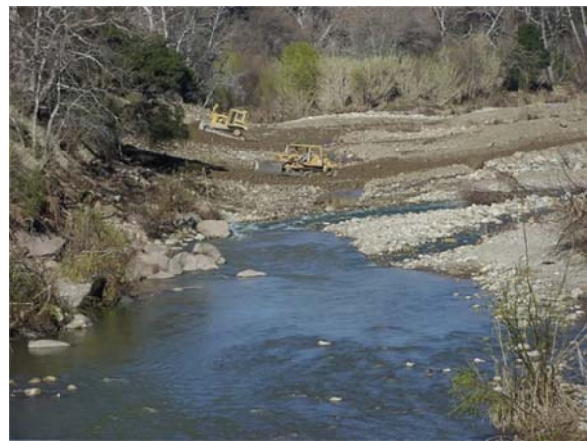
Flood Control Work – Ventura River
