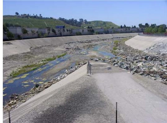
Flood Control—San Juan/Arroyo Trabuco Creeks
