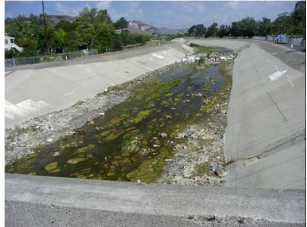
Channelization – San Juan/Arroyo Trabuco Creek
