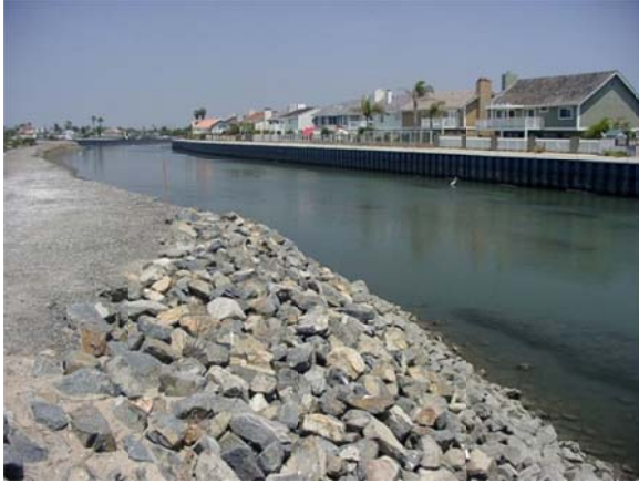
Wetland Fill - Santa Ana River Estuary
