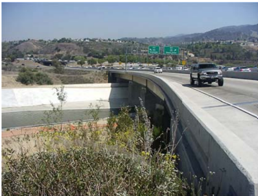
Urban Transportation and Flood Control
