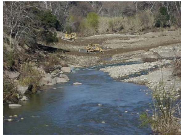
Flood Control Work – Ventura River
