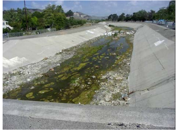
Channelization – San Juan/Arroyo Trabuco Creek
