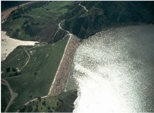
Twitchell Dam – Cuyama River
