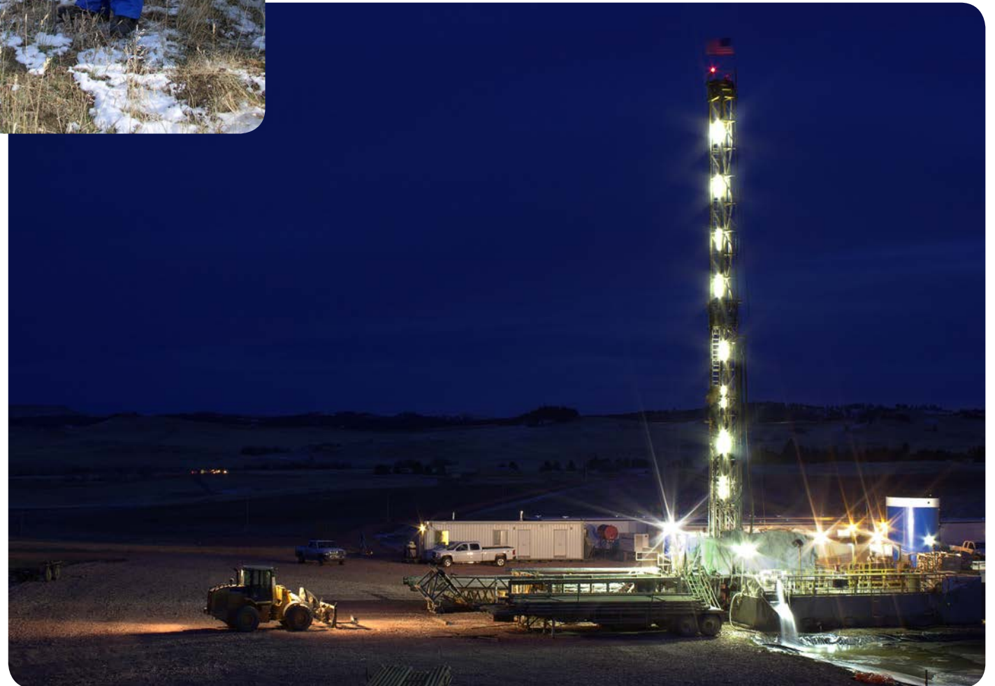
Drilling the observation well in the Bell Creek oil field.
