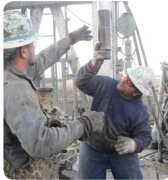
Core barrel retrieval on the drill rig.
