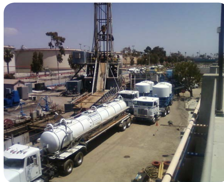
Drilling site in operation, during pumping and cementing activities.
