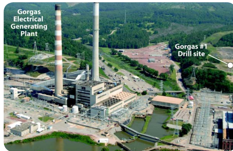
The William Crawford Gorgas Electrical Generating Plant, which is operated by Alabama Power Company, is one of two major coal-fired power facilities in the Black Warrior Basin of Alabama. The Gorgas #1 borehole was drilled near the power plant to investigate the potential for geologic carbon storage.
