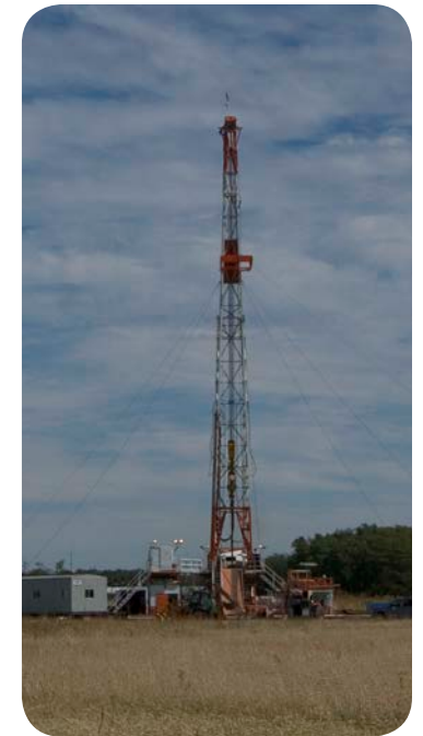
Spudding of Verification Well #1 at the IBDP site.
