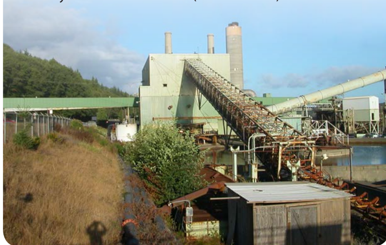
TransAlta's 1400 MW coal-fired power plant in Centralia, Washington.
