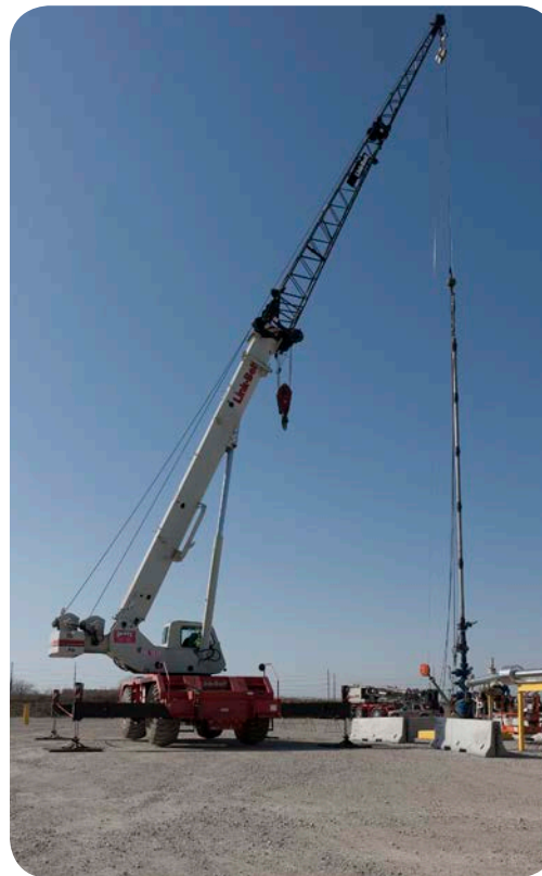
Logging of IBDP injection well concurrent with CO 2 injection.
