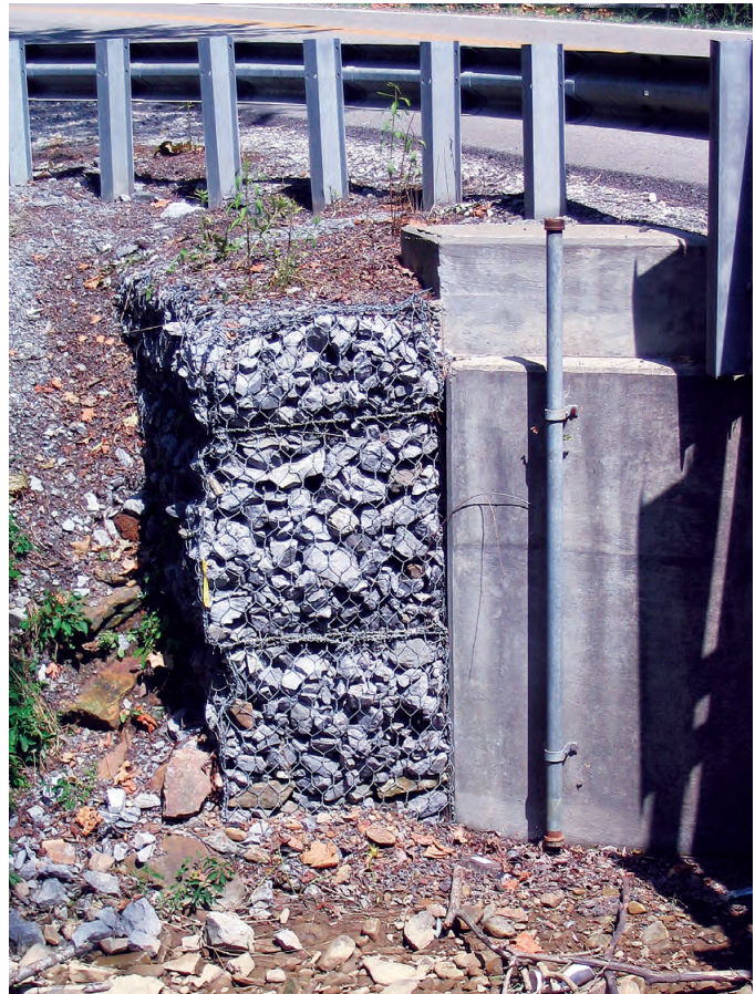
Figure 7. Crest-stage streamgage at Marsh Fork at Maben, West Virginia.
