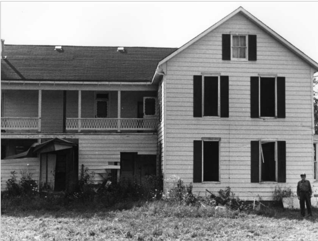
Figure 13.—Water barely reached to the first story of this house during the 1888 flood on the Cheat River. During the flood of November 1985, water reached the second floor.
