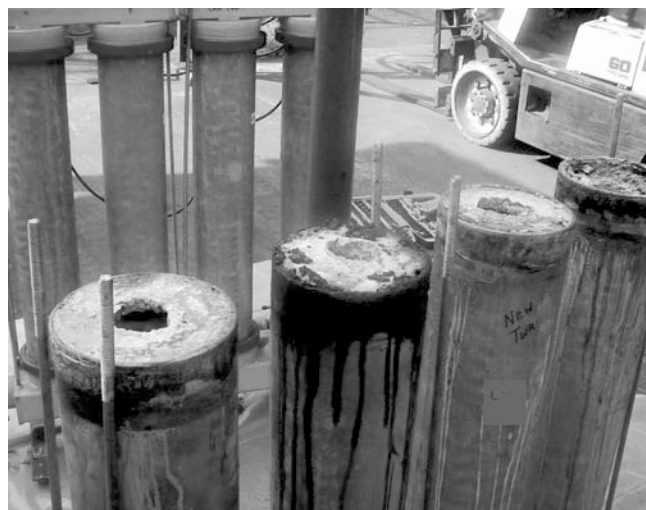
Figure 3 8 inch cells used to treat 450 ton industrial cooling tower under zero discharge mandate.
