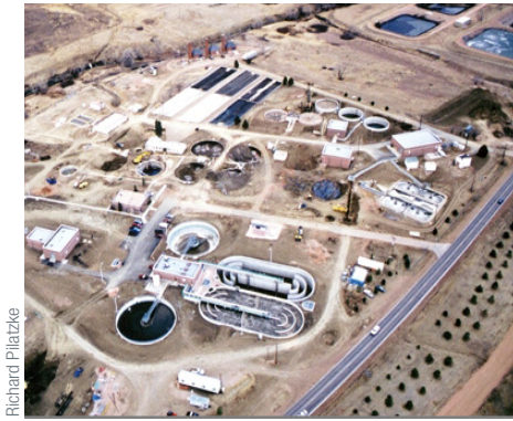
Figure 2. Reclaim Water at Fort Carson.
