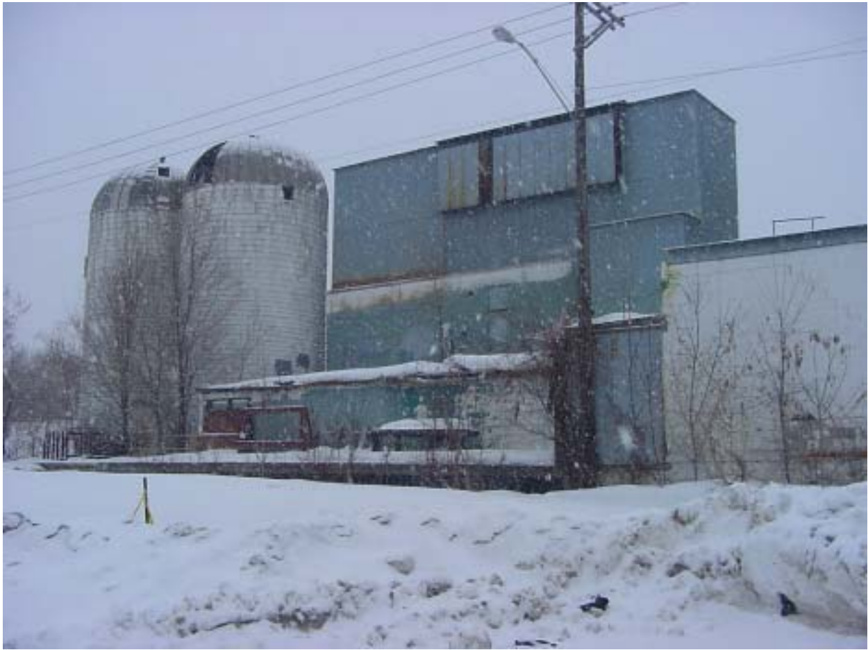
Figure 1. Photograph of the Western Mineral Products/W.R. Grace facility taken in February, 2001. This photo shows the north side of the four-story, sheet-metal building that housed the expanding furnace. To the left are raw material storage silos, and to the right is the cement-block building for product handling and shipping.
