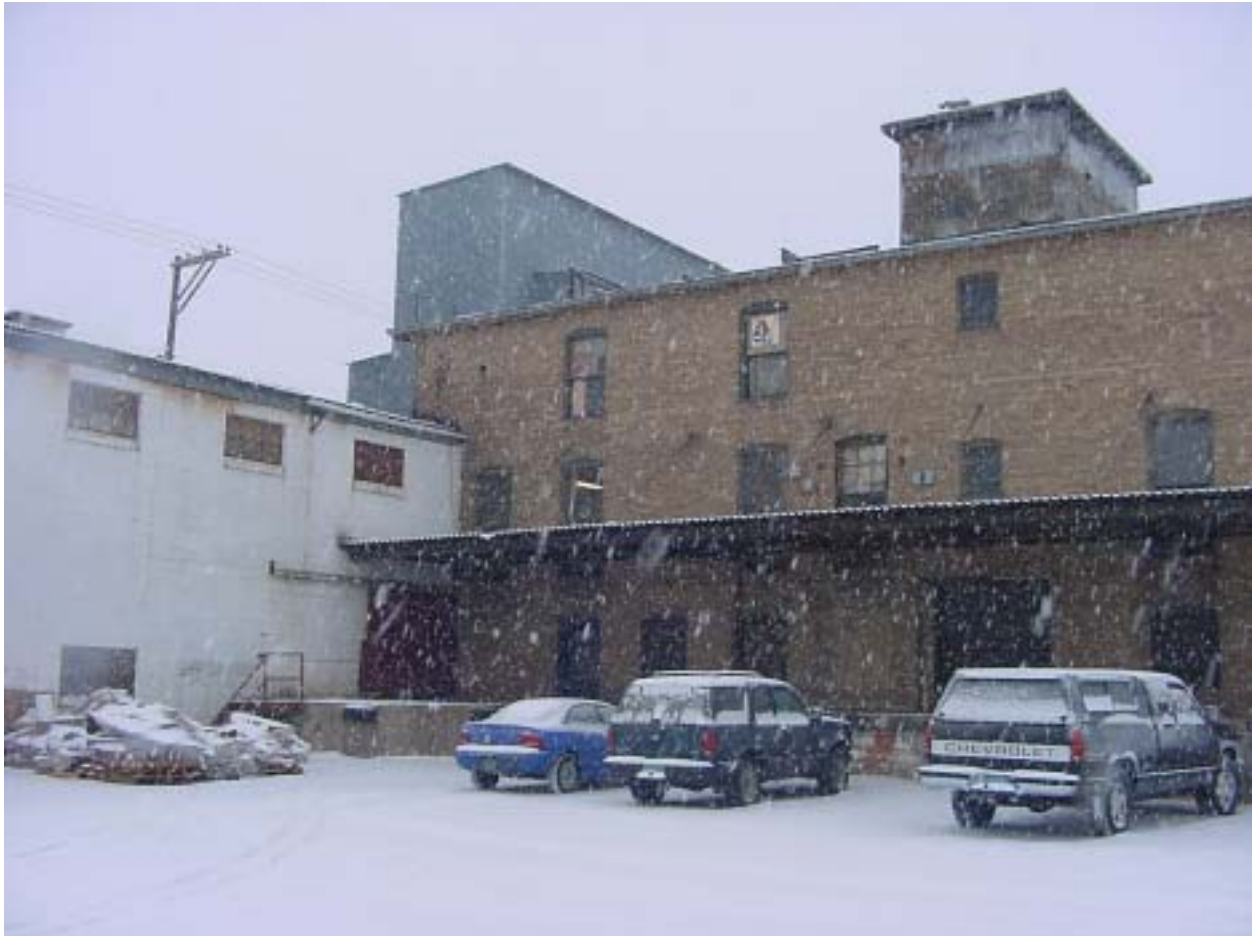
Figure 2. Photograph of the Western Mineral Products/W.R. Grace facility taken in February, 2001. This photo was taken from the southwest side of the facility. The four-story, sheet-metal building that housed the expanding furnace can be seen in the background. To the right is the brick building which housed operations and some shipping, and to the left is the cement-block building for product handling and shipping. The waste pile was located at the far left end of the cement-block building.
