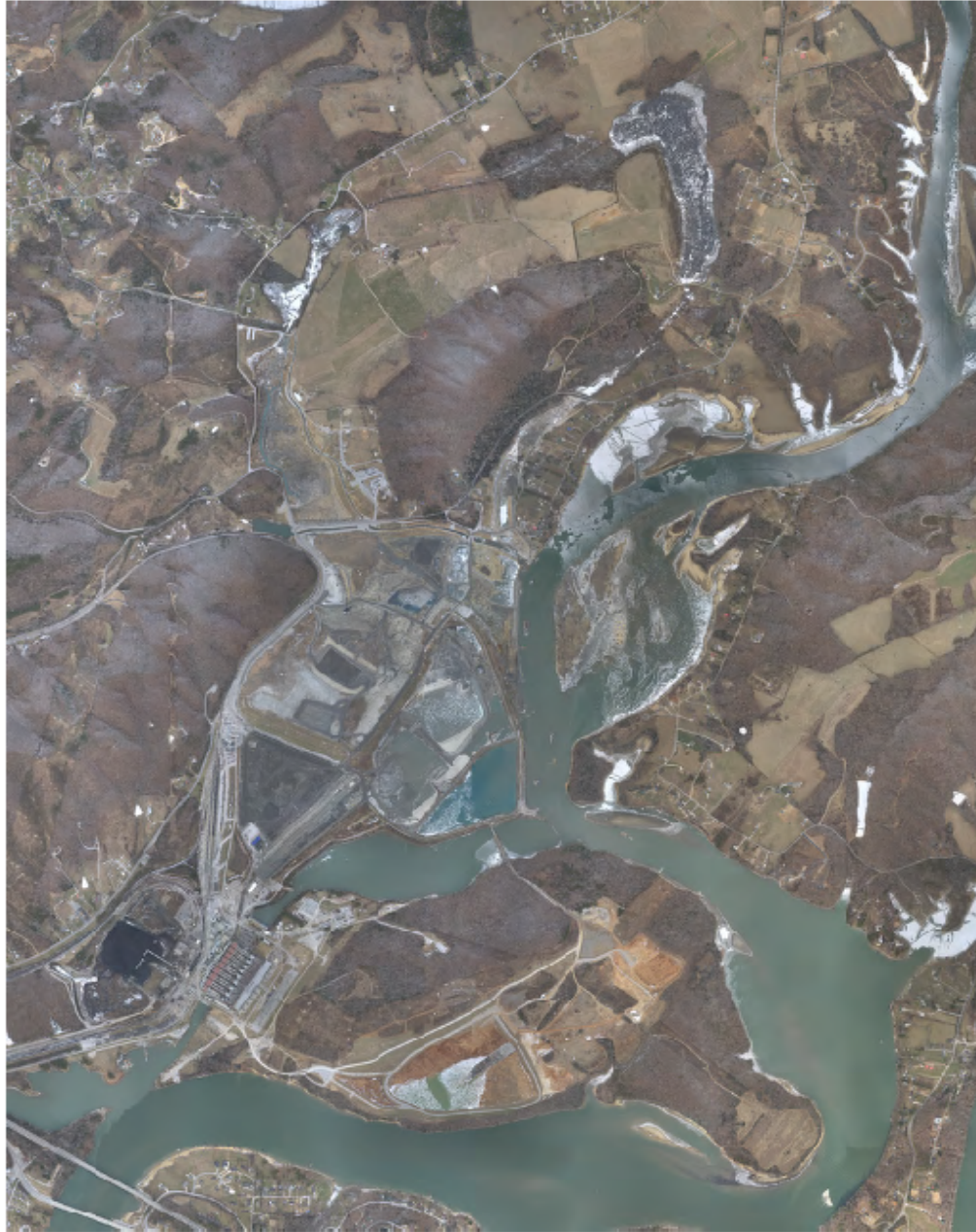
Aerial Image of Kingston Ash Slide (01/11/2010)
