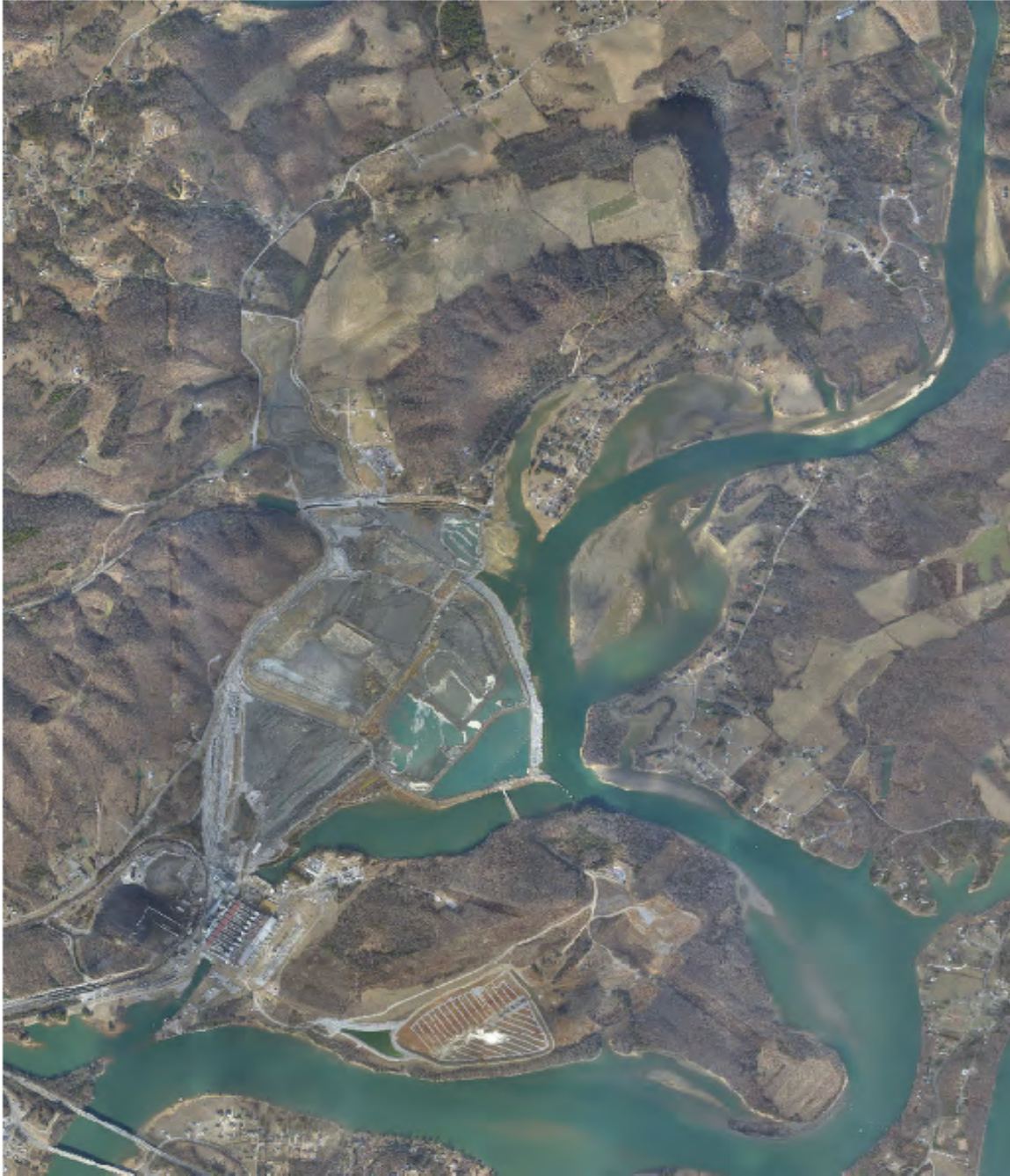
Aerial Image of Kingston Ash Slide (01/24/2011)
