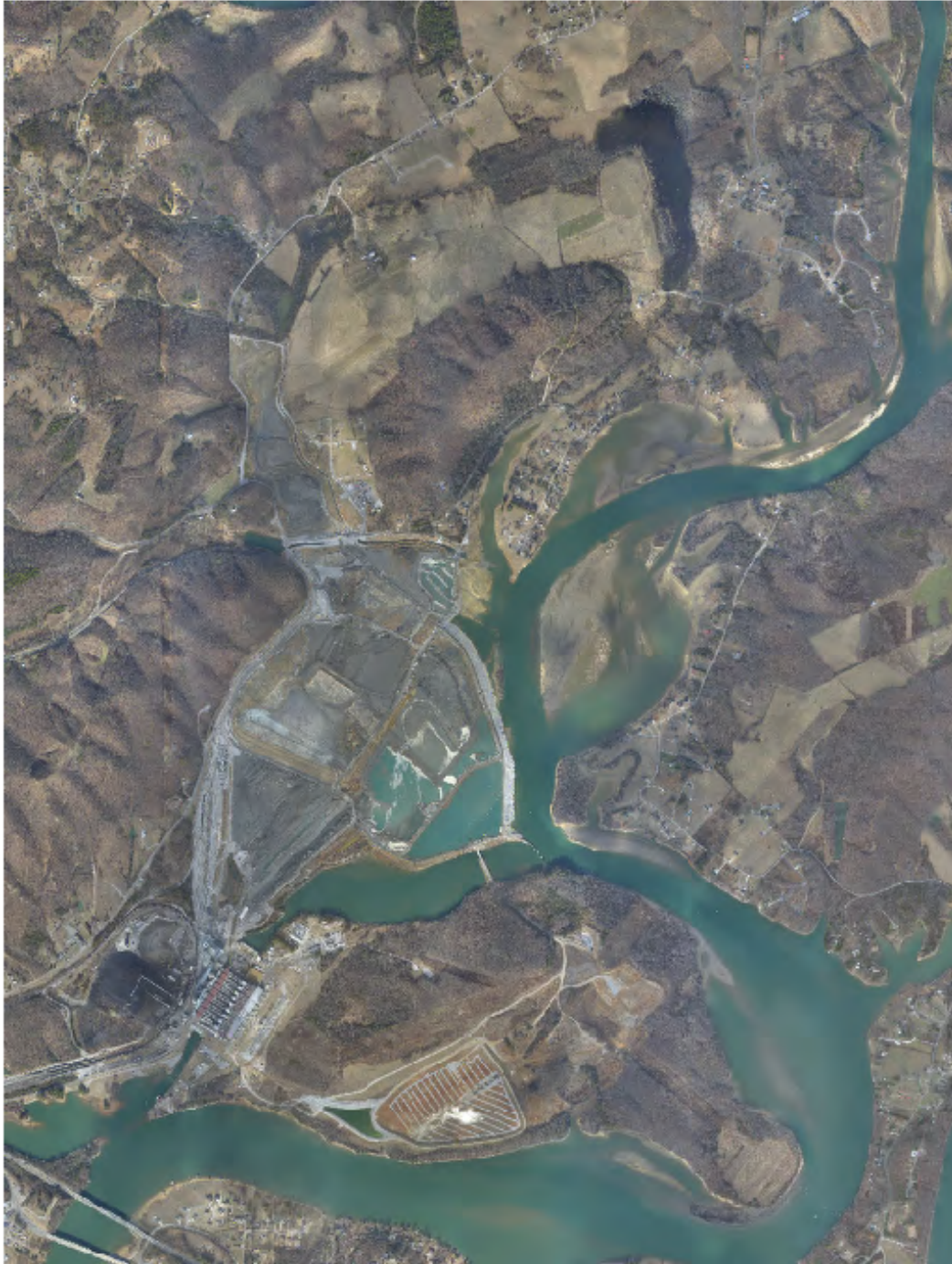
Aerial Image of Kingston Ash Slide (01/24/2011)
