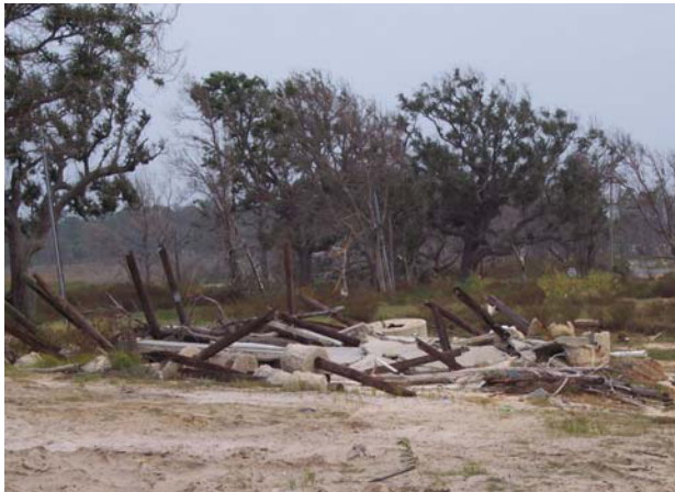
Figures 31, 32, 33, and 34. Failed Supporting Foundations
