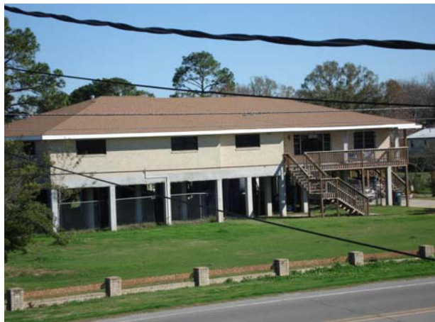
Figures 35, 36, and 37. Segmented Piles Construction Method
