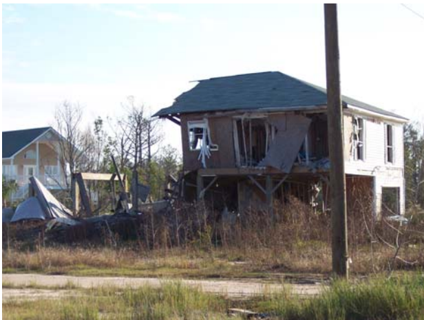
Figures 10, 11, 12 and 13. Damages to Elevated Structures
