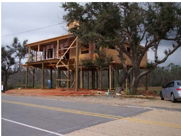
Figures 22, 23, 24, and 25. Open Foundation Types
