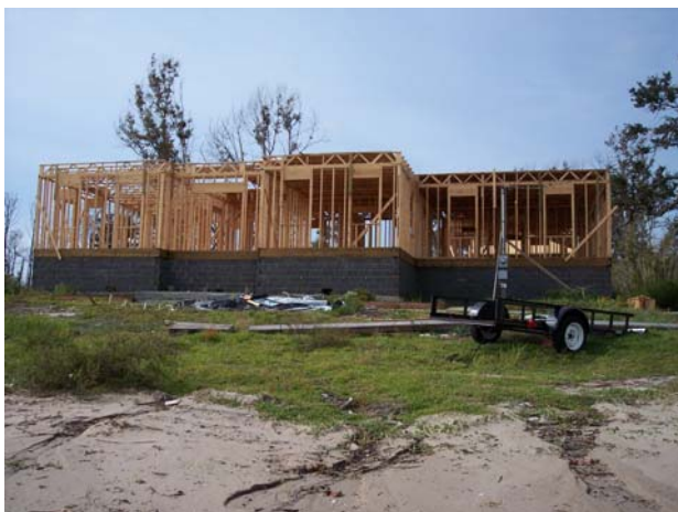
Concrete Block Enclosure
