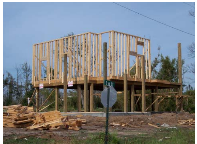
Wood Post and Piling
