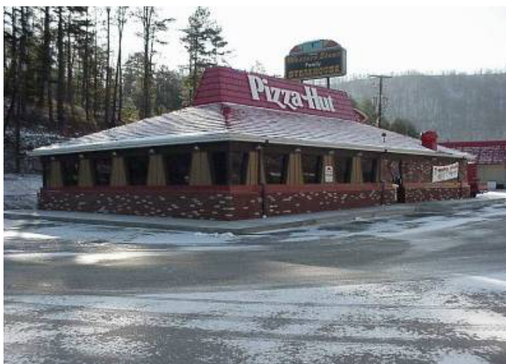
Figure 48. Veneer Wall Installation
