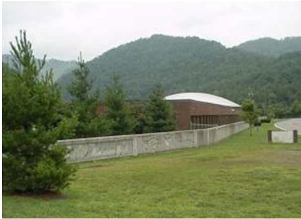
Figure 49. Ringwall Protection for a High School
