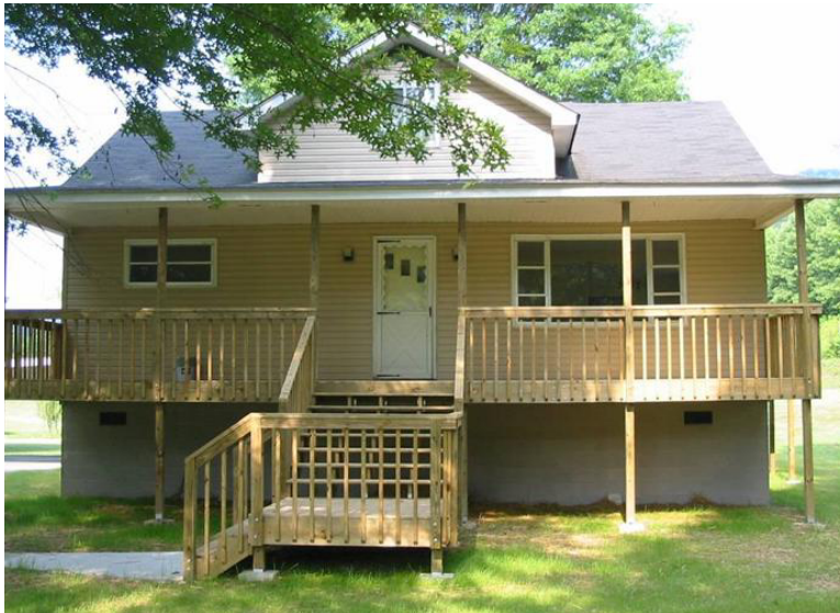
Figure 26. Structure Raised on Solid Wall Foundation
