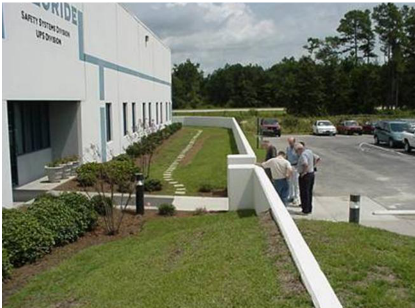
Figure 50. Ringwall Protection for a Commercial Structure
