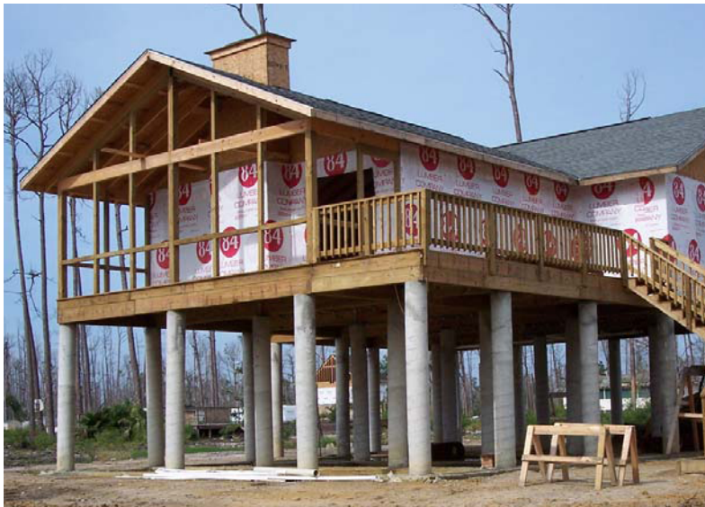
Figures 40 and 41. New Concrete Column Construction
