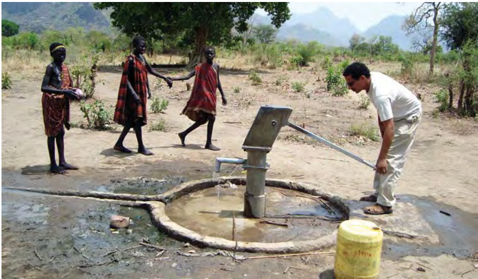
Testing the handpump of a borehole in Eastern Equatoria, Southern Sudan.
