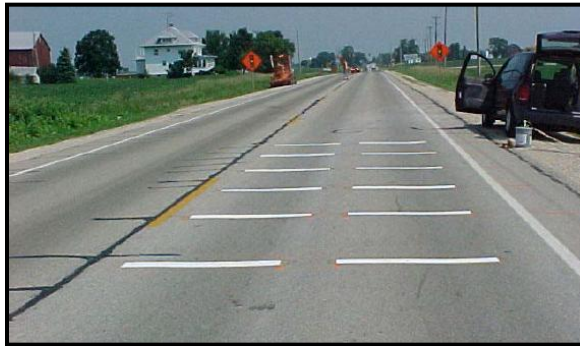
FIGURE 2.2 The installation of rumbler (Horwitz 2002)
