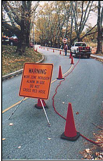
FIGURE 2.4 The installation of pneumatic tube intrusion alarm (Hatzi 1997)
