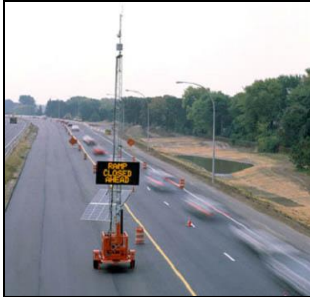
FIGURE 2.16 Integrated PCMS and HAR systems in a work zone (FHWA 2010)
