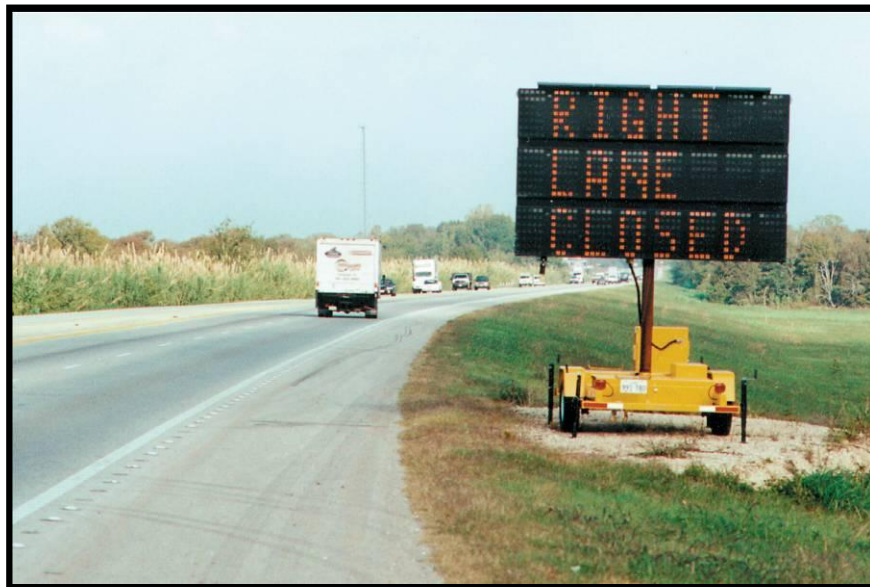
FIGURE 2.6 The installation of a portable changeable message sign in Texas (Texas Transportation Institute 2004)
