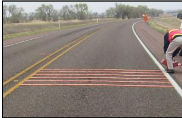
FIGURE 2.1 The installation of orange rumble strips (Fontaine 2010)
