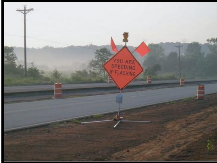
FIGURE 2.8 The installation of vehicle activated sign (Mattox III et al. 2007)
