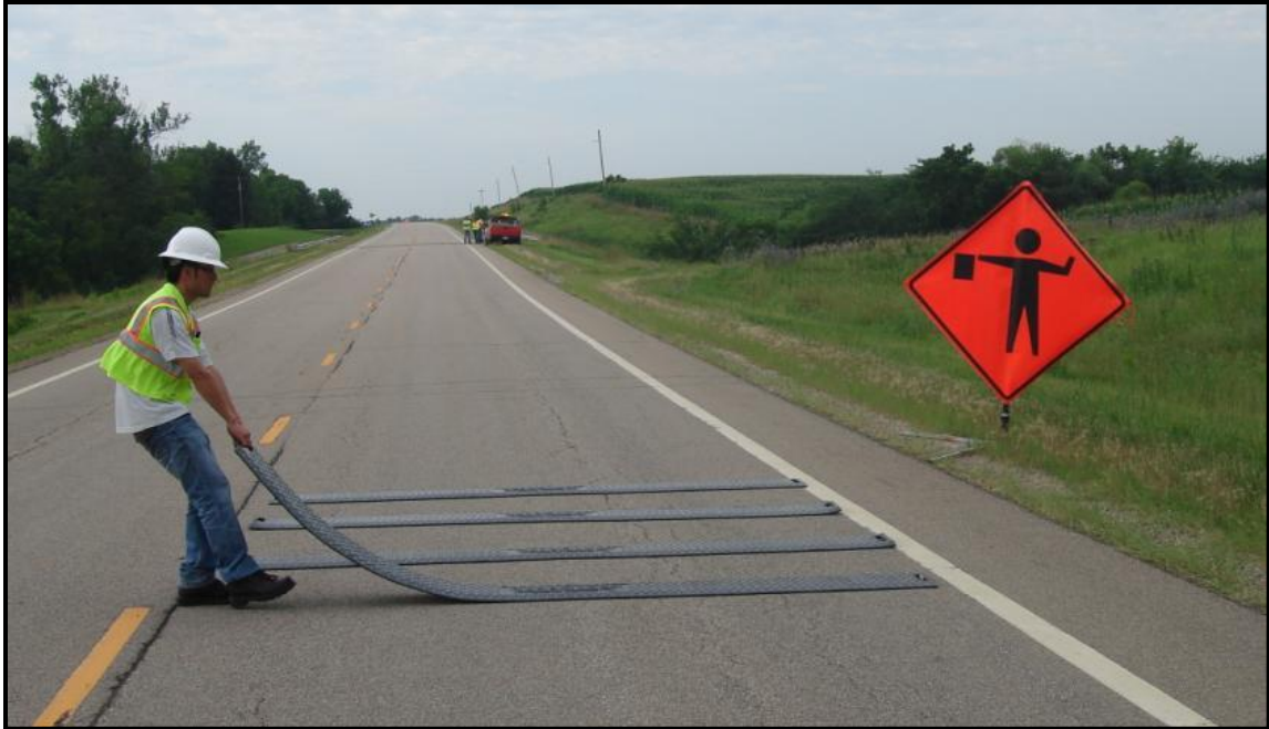
FIGURE 4.3 Installation of PPRs at Site 1
