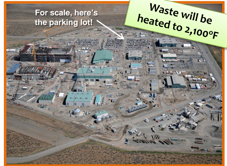
Aerial view of construction, July 2011
