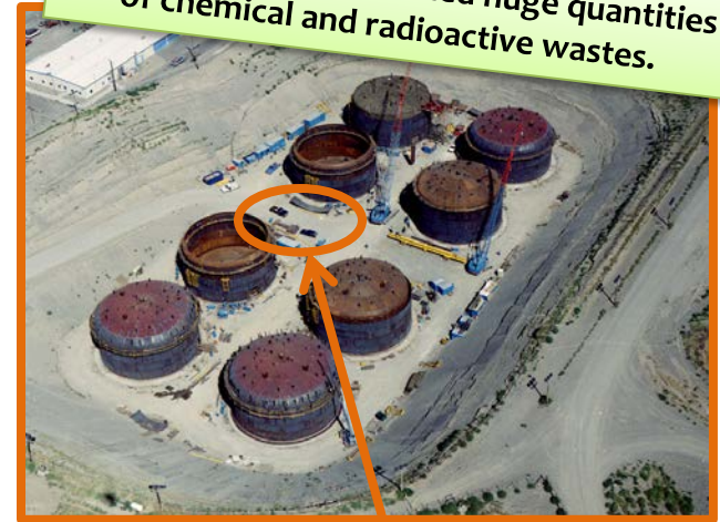
241-AP Tank Farm construction. See black pickup trucks for scale.
