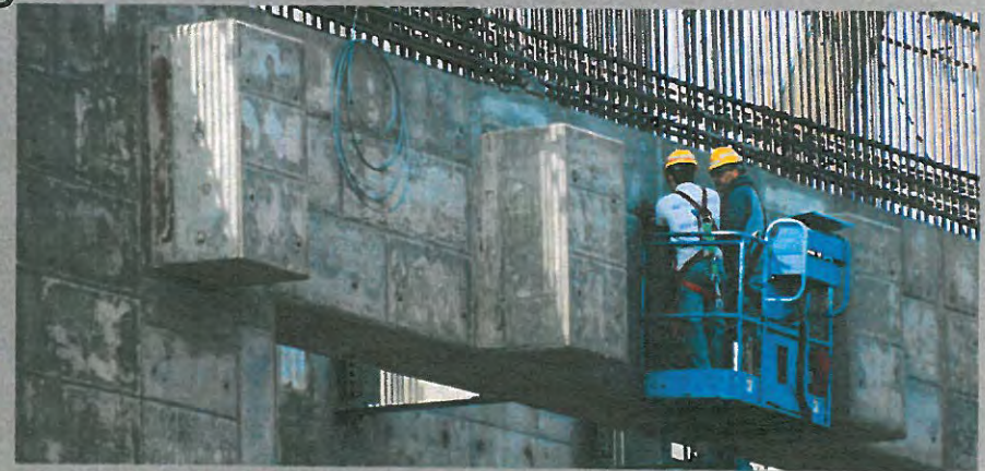
High-Level Waste Facility truck bay walls
