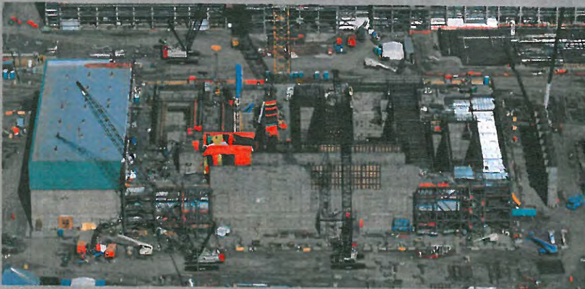
High-Level Waste Facility exterior
