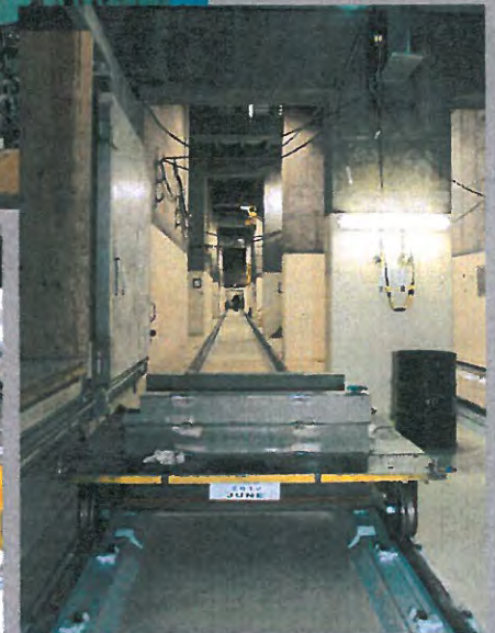
Low-Activity Waste transfer tunnel
