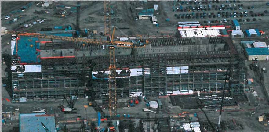
Pretreatment Facility exterior
