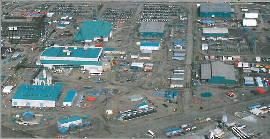
18 support buildings for the Balance of Facilities
