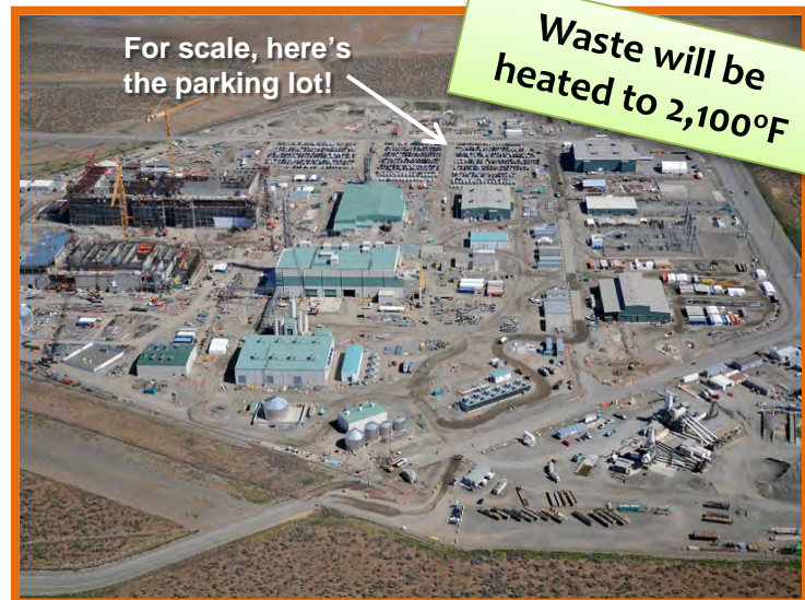
Aerial view of construction, July 2011
