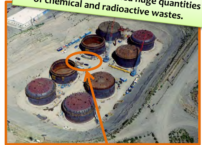
241-AP Tank Farm construction. See black pickup trucks for scale.
