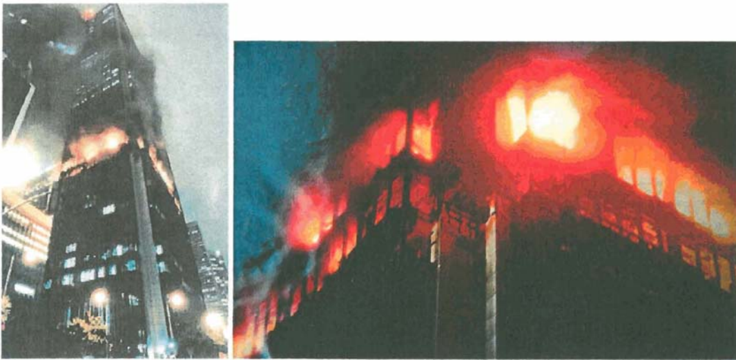
Figure 1 First Interstate Bank Building, Los Angeles, May 14, 1988
