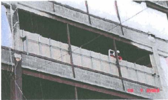
Figure 4 Cardington Facility Test Interior Columns
